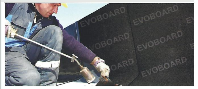
EVOBOARD is a tough semi-flexible, rot-proof durable pre-molded bitumen board suitable for a variety of applications in below or above ground waterproofing as well as roofing, parking, bridge decks, wet areas, planters, pools, fountains and civil works.
